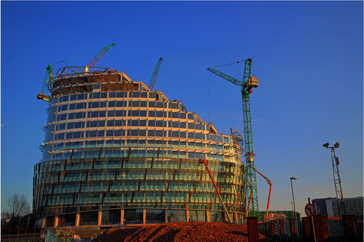
Fig. 2 Construction of the double skin façade at One Angel Square, Manchester, UK [source: Alastair Wallace / Shutterstock.com]
