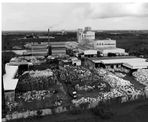
Figure 1: SMC Solid Waste Infrastructure Collection Plant
