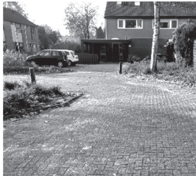
Figure 2. Impression of the local situation at Griffiersveld in the municipality of Apeldoorn, before reconstruction took place.
